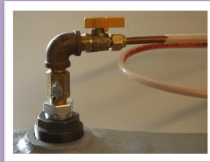
Top Feed HFOSV-12 Valve (Anti-Siphon)
